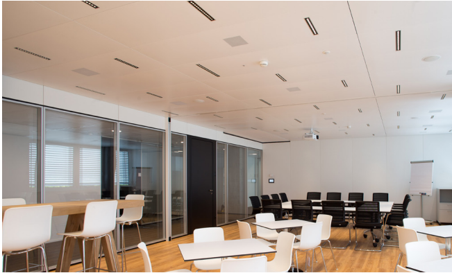
Heiz- /Kühldecke Metall
