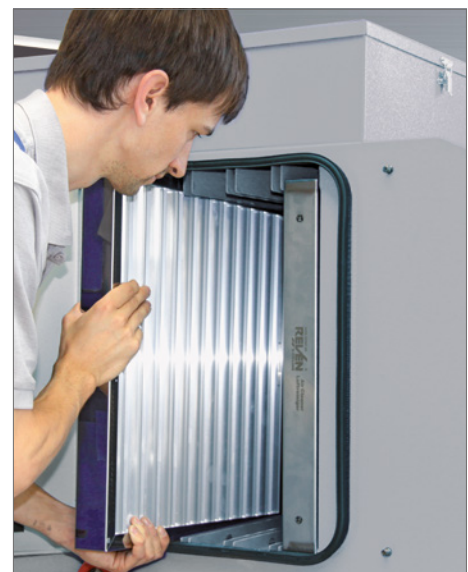
Fig.: When installing the filter, the profiles must be arranged vertically.
